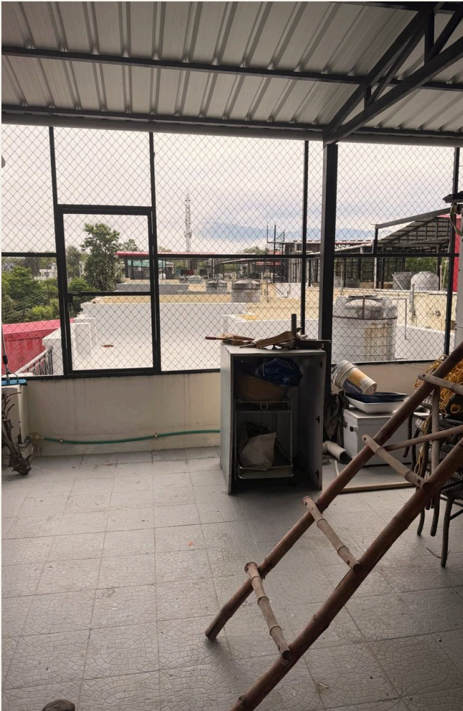
BEFORE · A MESH ENCLOSURE UNDER A SHEET ROOF, USED FOR STORAGE
